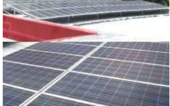
Pertamina Gasoline Station - Cililitan Jakarta
