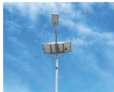
Rest Area Toll Palikanci KM 207 A - Cirebon
