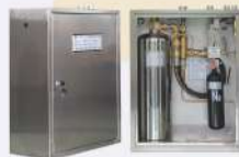
Kitchen wet system
